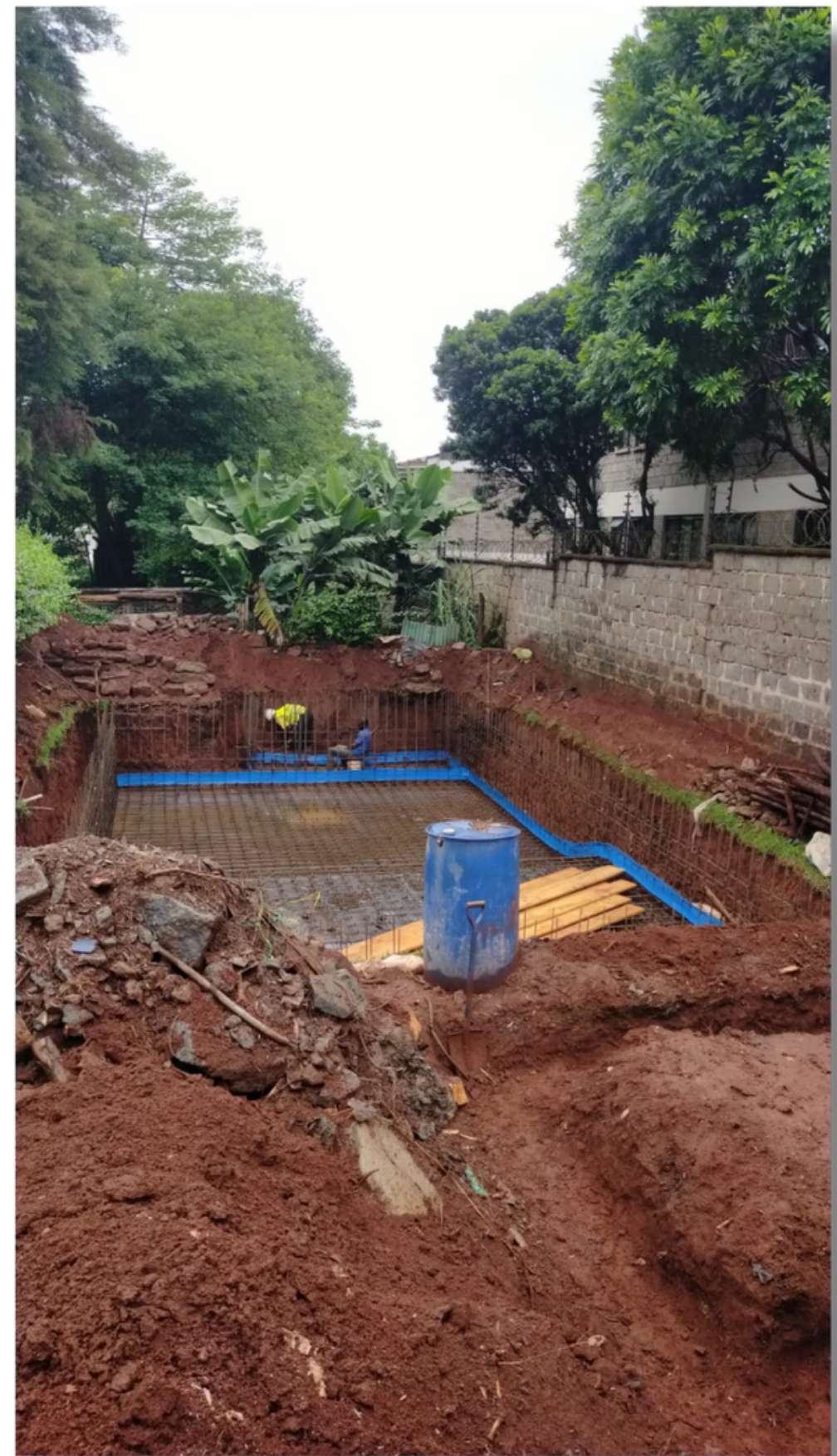
A Swimming Pool under construction at a Residential Premise in Nairobi.
