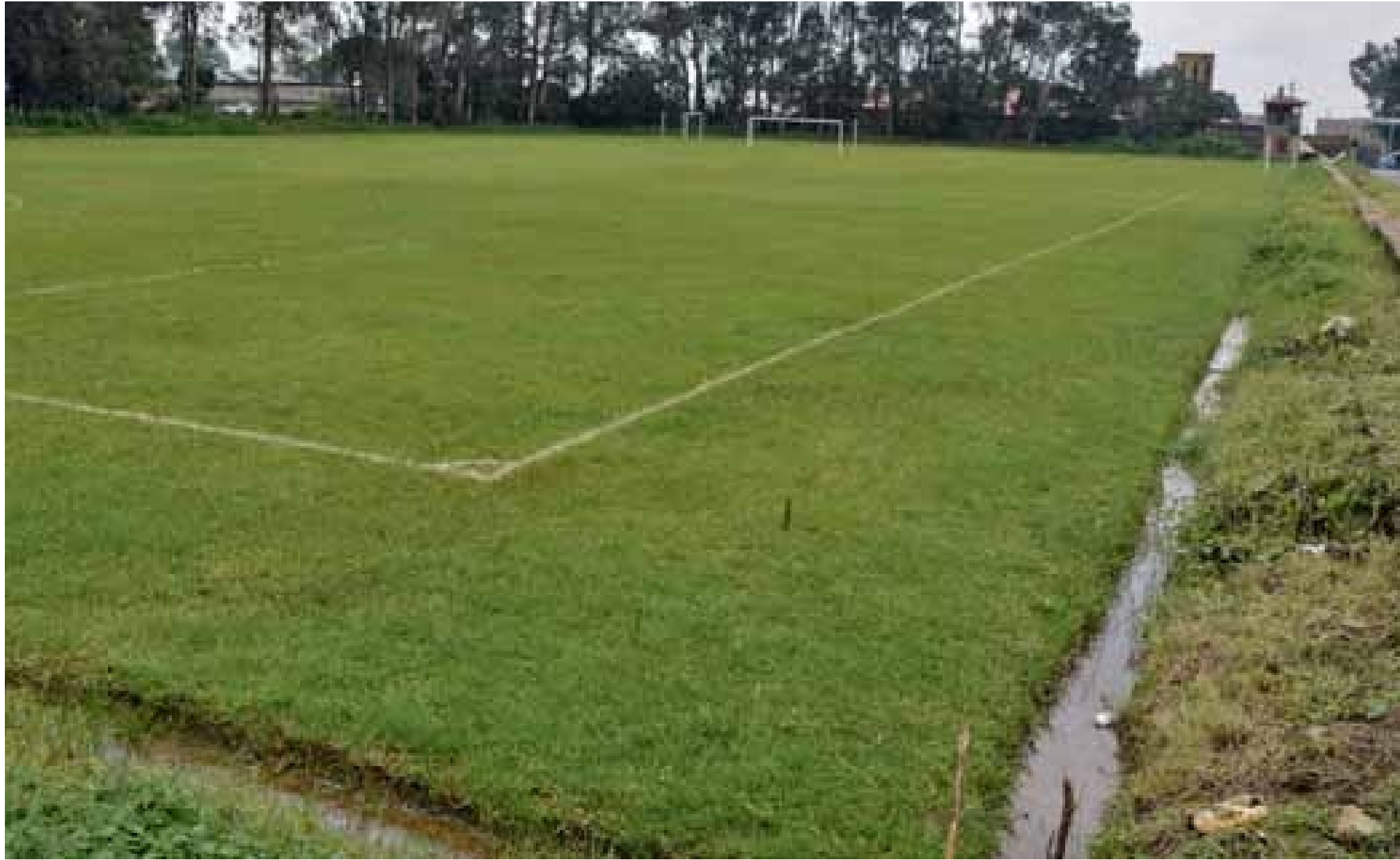
Natural earth channel (drainage type 1) filled with excess water at a Polytechnic College.
